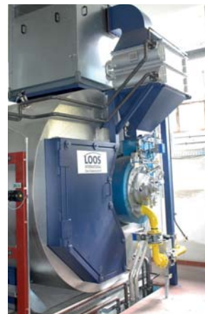
The RAY industrial gas burner with air preheater for the utilization of waste heat from compressors
