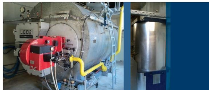
Increased efficiency: The new firing with speed regulation and oxygen control as well as the retrofitted economizer
