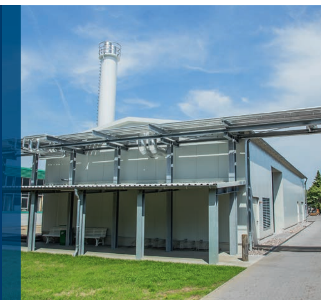
Exterior view of Valenzi's boiler house
