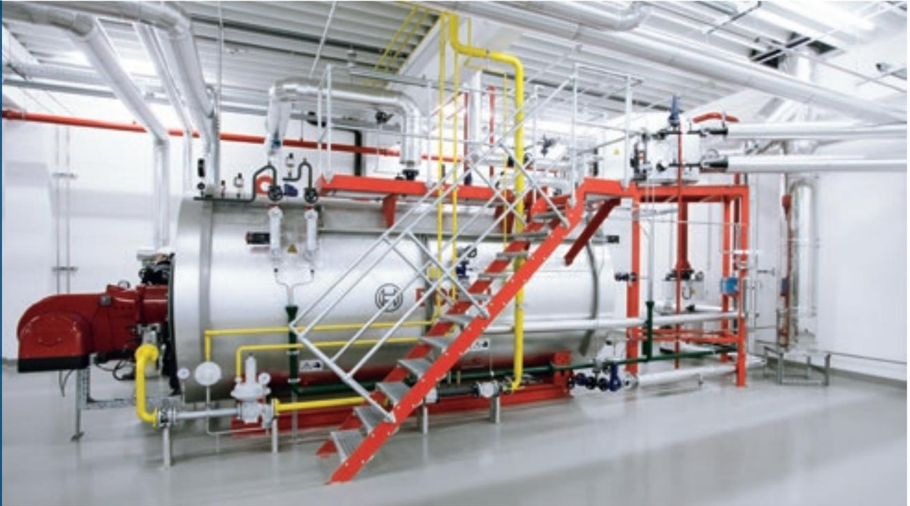
The new, highly efficient UL-S steam boiler fired with natural gas and heat recovery equipment
