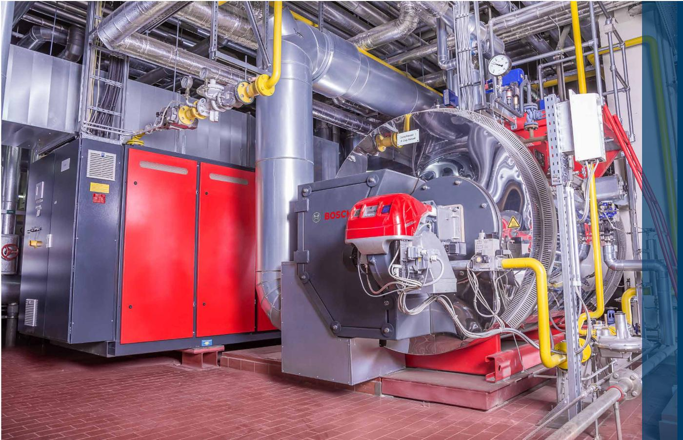
Effective use of waste heat sources: The CHP waste heat with temperatures of up to 550 °C are passed through the fourth pass of the steam boiler and used for the steam generation.
