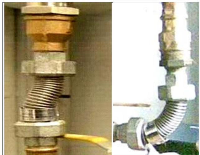
Fig. 1 Examples of axial compensator bad installation practice
