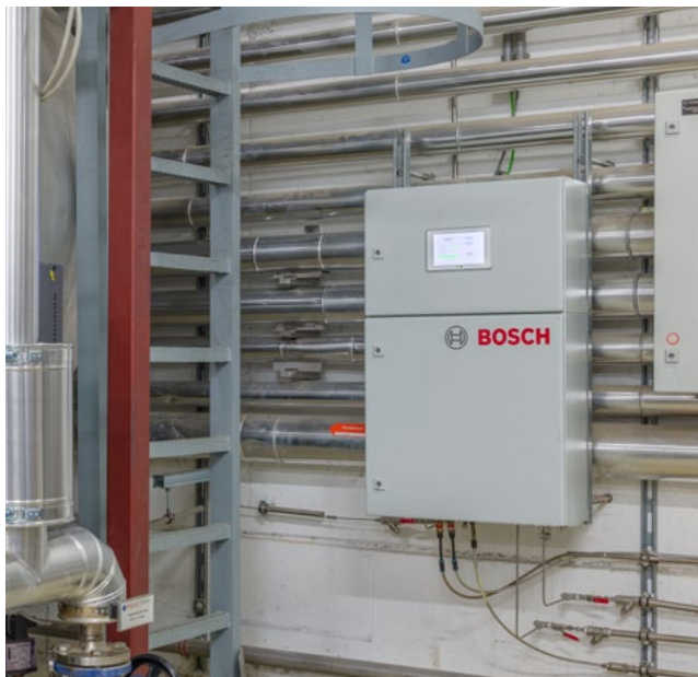
Fully automatic and reliable: The space-saving module continually checks the relevant water parameters.
