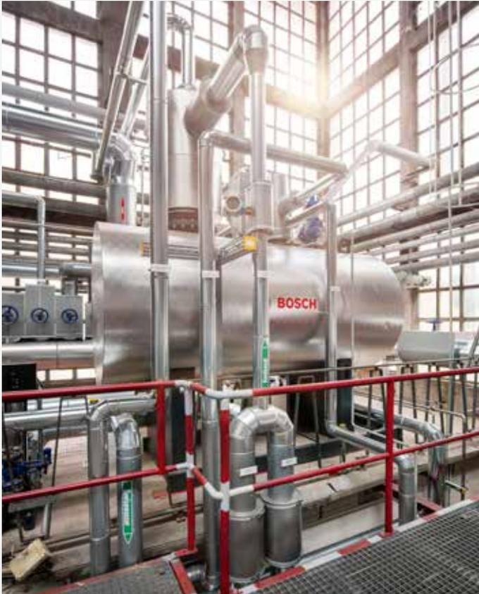
*The feed water deaeration system was placed one floor higher in Pirmasens. Heating the feed water to 103 °C ensures that corrosive elements in the feed water dissolve. To make the process more efficient, a downstream vapour cooler uses accumulating exhaust vapour to pre-heat make-up water.*
