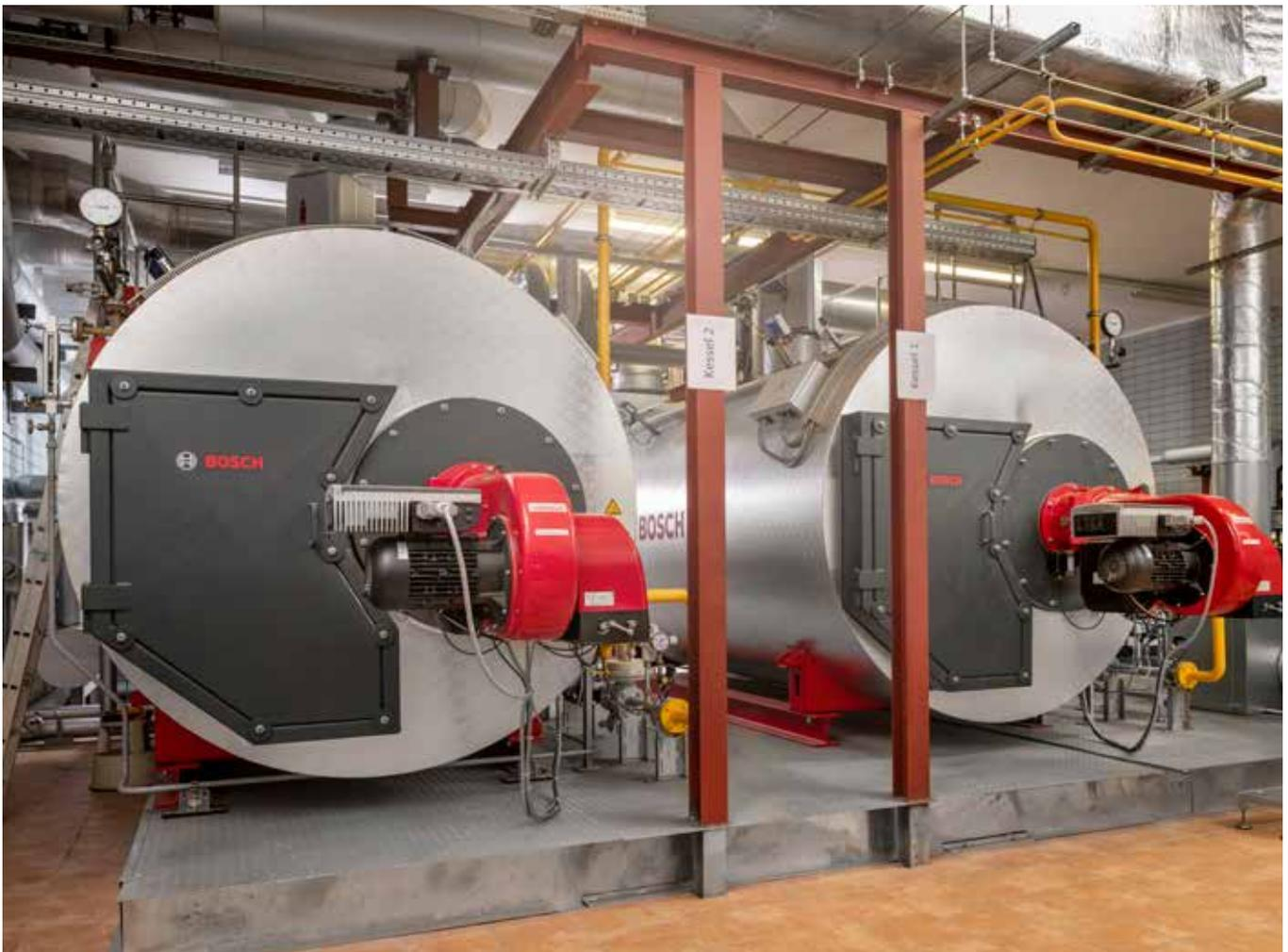
*The Bosch boilers in Bellheim supply the brewery for processes like mashing and boiling. A cascade control ensures exceptionally cost-effective operation of the multi-boiler system.*
