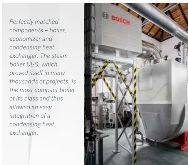
*Perfectly matched components – boiler, economizer and condensing heat exchanger. The steam boiler UL-S, which proved itself in many thousands of projects, is the most compact boiler of its class and thus allowed an easy integration of a condensing heat exchanger.*
