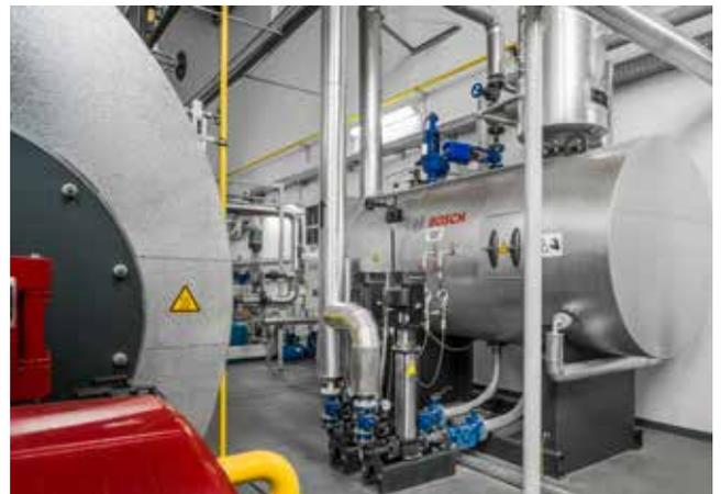
*The deaeration module from Bosch protects boiler and components from corrosion and increases operating safety. The module is delivered pre-assembled from the factory and can be installed within shortest time.*
