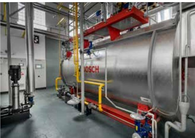
*Demand-oriented and fully automated: Reduced obligation to supervise with cold start automatic as well as automatic desalting and blow-down for an efficient operation.*
