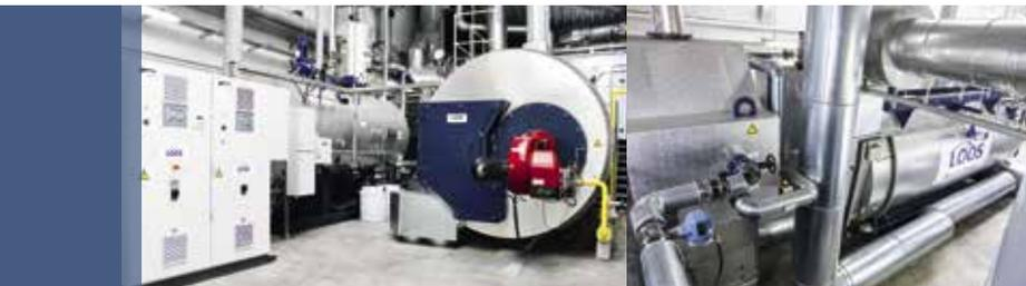
In addition to the four-pass boiler, the system also includes modular components for water treatment and heat recovery from Bosch Industriekessel.
