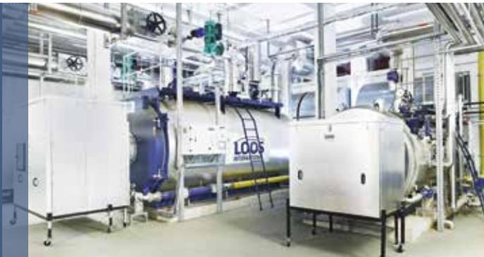
Efficient supply of heat and steam: The UT-L heating boilers as well as one UL-S steam boiler.
