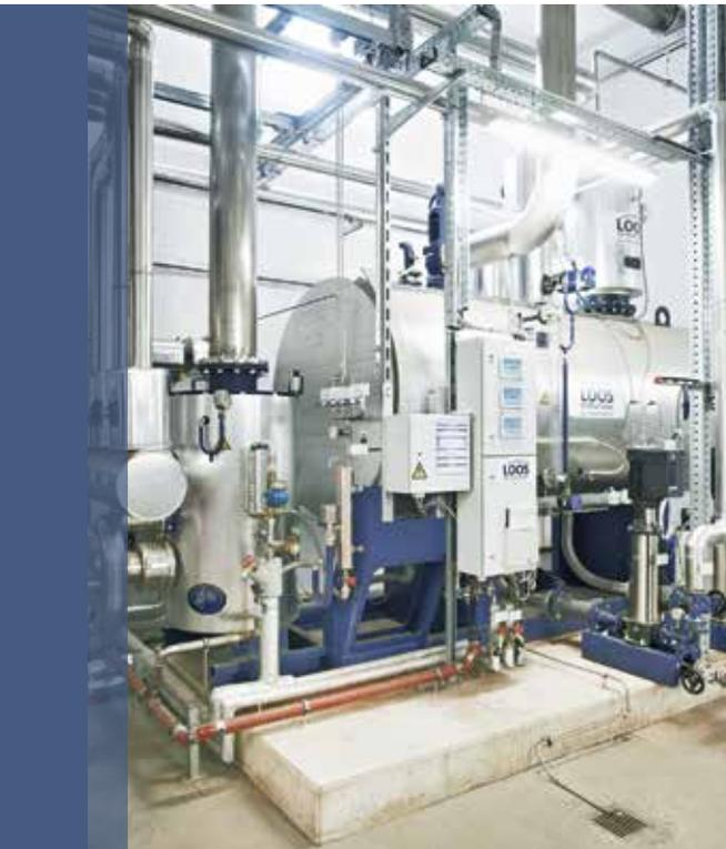
The water service module WSM-V ensures fully automatic water treatment. The main components of the module are a steam-heated feed water tank with trickling deaerator, chemicals dosing device, blow-down and expansion tank, a water sample cooler as well as a modern control panel. The WA water analyser ensures optimum water quality.
