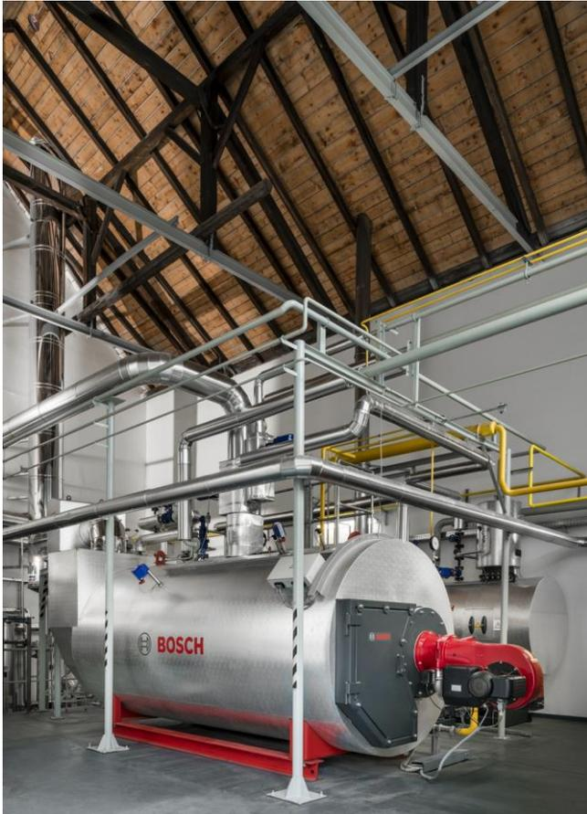
The steam boiler UL-S from Bosch efficiently supplies brewhouse, bottle and keg cleaning with steam.
