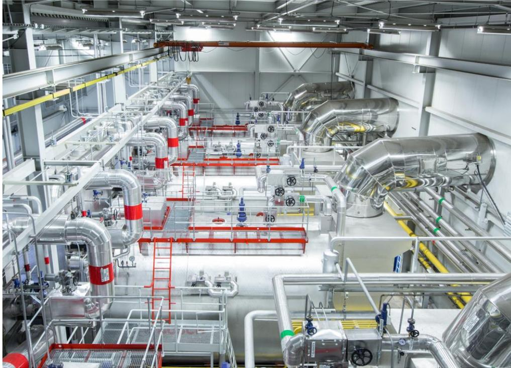
The boilers can produce up to 167 tons of superheated steam per hour for starting up the steam turbine and supporting the district heat supply.
