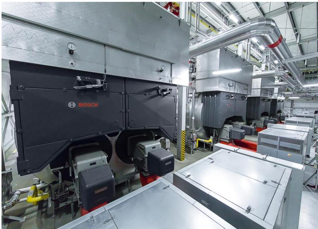
Each of the boilers are equipped with two natural gas burners, both single and parallel operation is possible.
