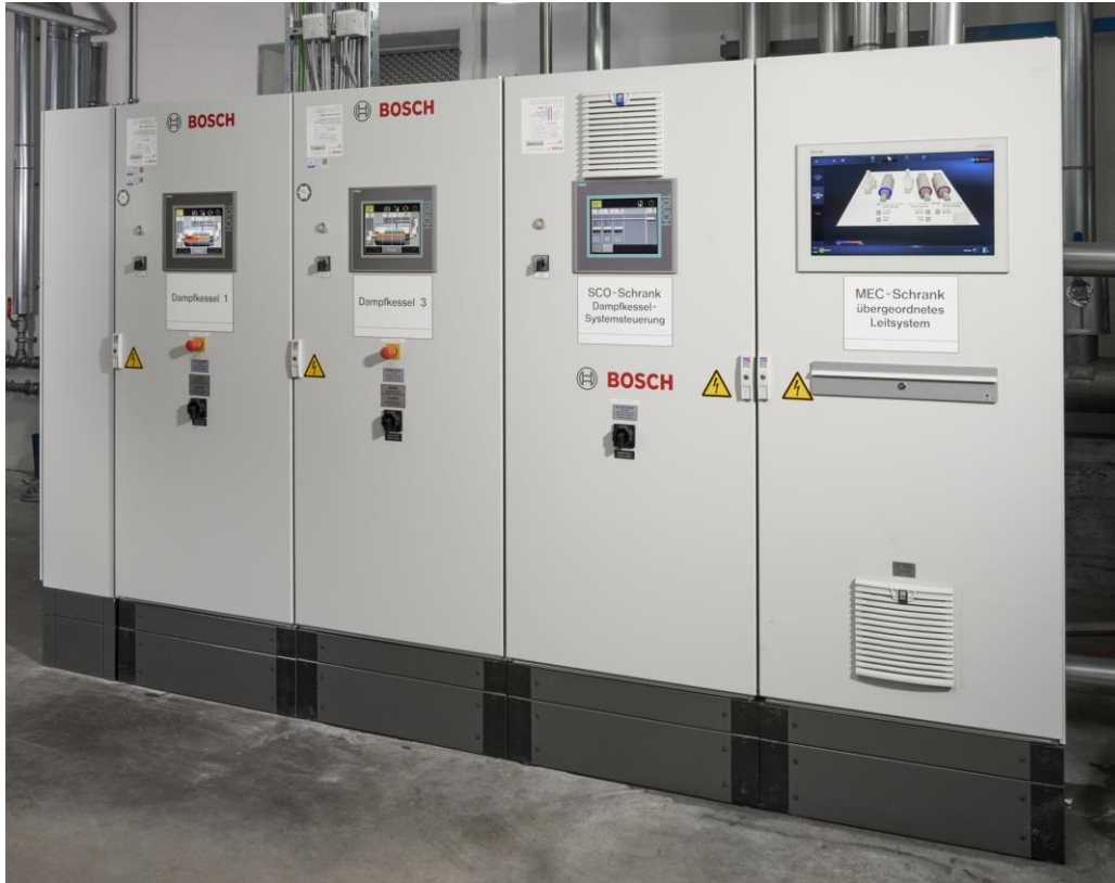
The new boiler and system controls with superordinate control system Master Energy Control from Bosch.
