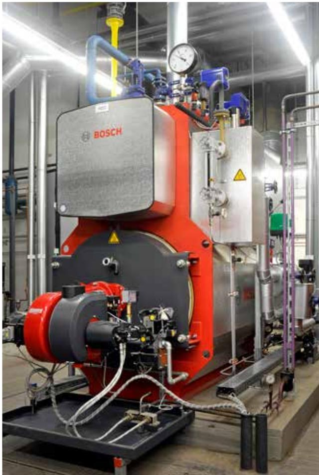
*The compact steam boiler U-MB with an economizer and natural gas firing.*
