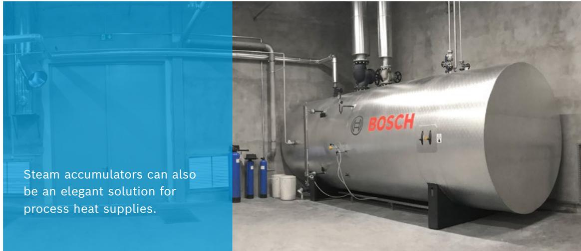
Steam accumulators can also be an elegant solution for process heat supplies.
