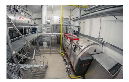
Figure 8: Hans Heinglein und Sohn GmbH's particularly efficient steam boiler system with an integrated economiser and downsteam flue gas condenser.
