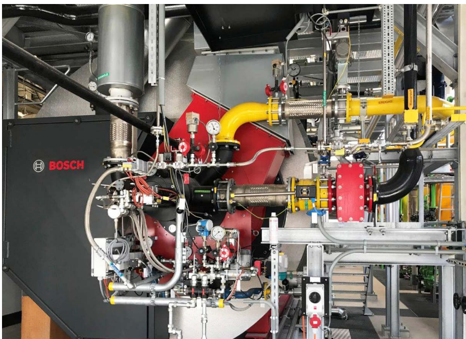
Fig 4: Example of an implemented fuel concept with hydrogen, natural gas and light fuel oil for a Bosch boiler system at a pharmaceutical company.
