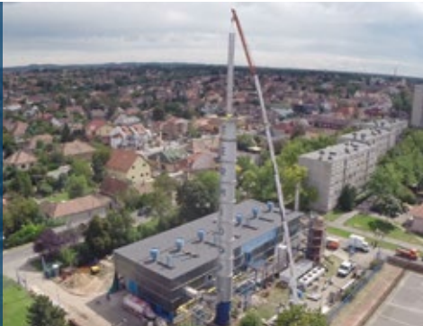
Dunakeszi Közüzemi Kft. heating plant during the rebuilding phase
