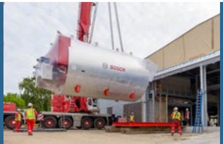
Delivery and positioning – each boiler had a transportation weight of 68 tons
