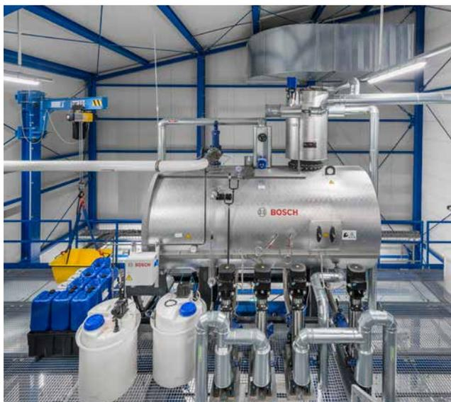
The water service module (WSM) is installed on the second level in the boiler house and provides the boilers with thermally-treated feed water.
