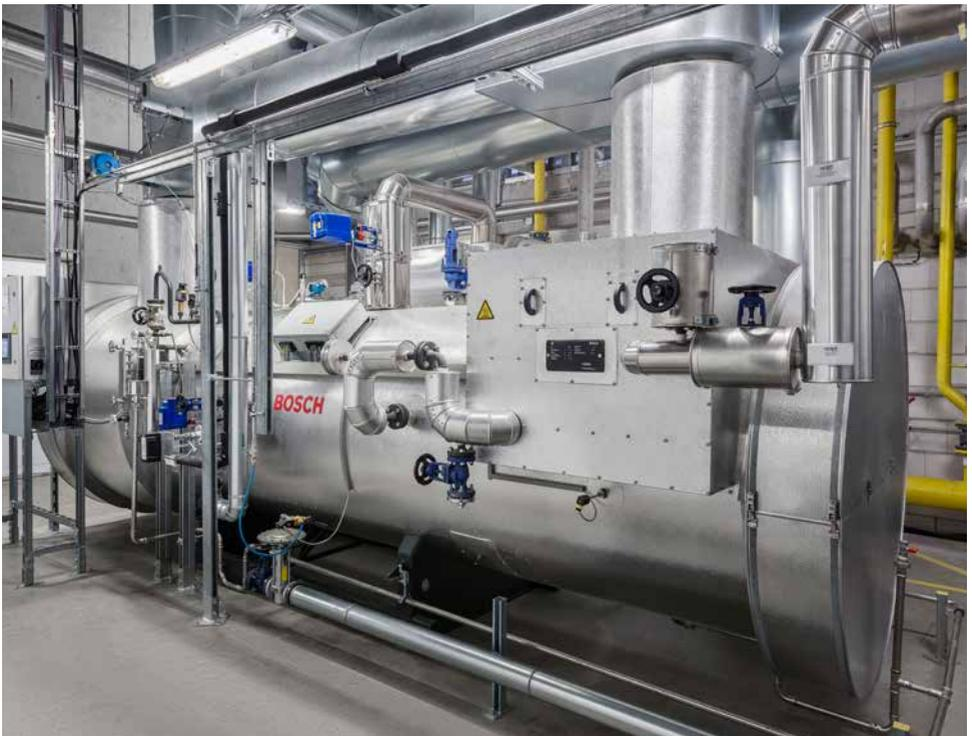
High-efficiency and resource-saving: The HRSB uses the waste heat from the CHP engine to generate steam.
