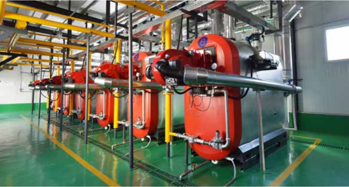
Extremely low NO x emissions: The optimised Uni Condens boilers with recirculation technology.
