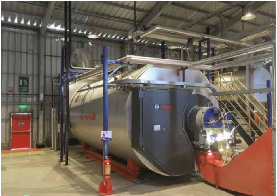
Powerful and highly efficient: the UL-S steam boiler can provide up to 20 t/h of steam for producing hygienic paper products.
