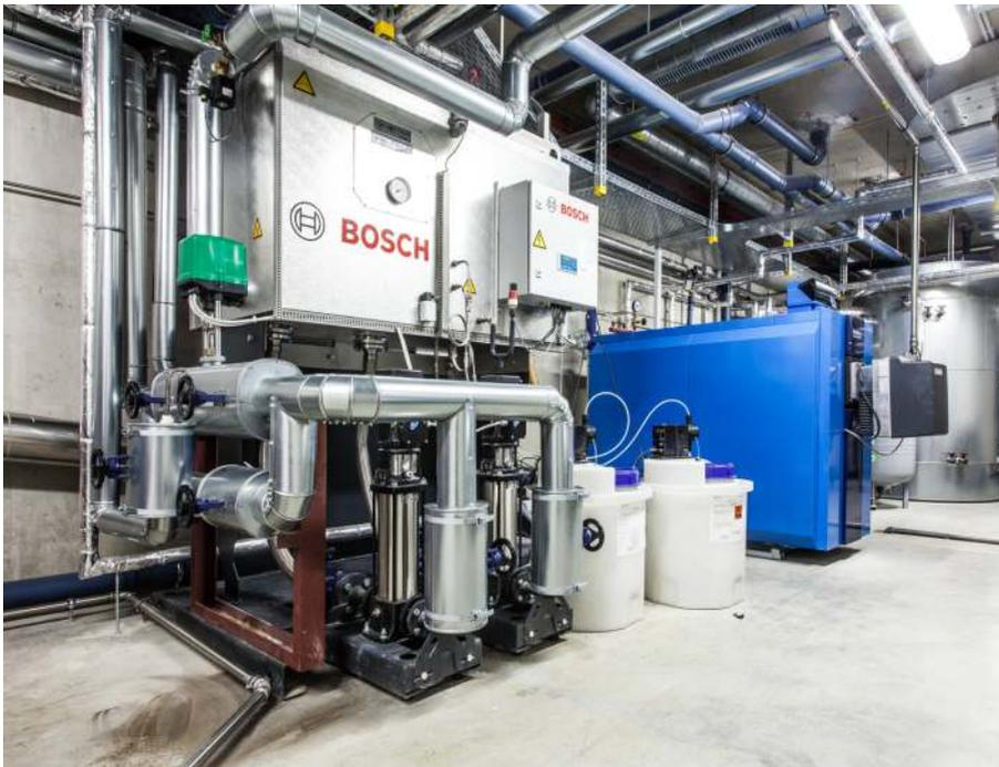
Boiler system automation and intelligent system control reduce energy losses and the internal consumption of the system.
