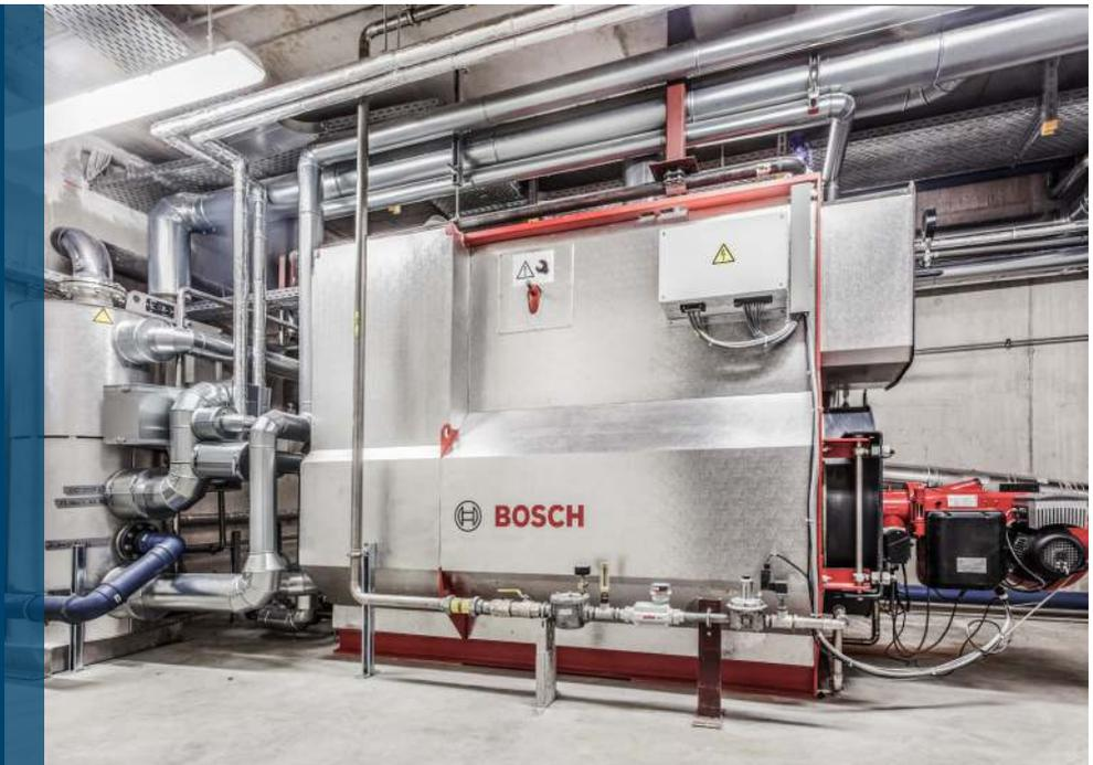
The boiler type U-MB impressed with its compact design.
