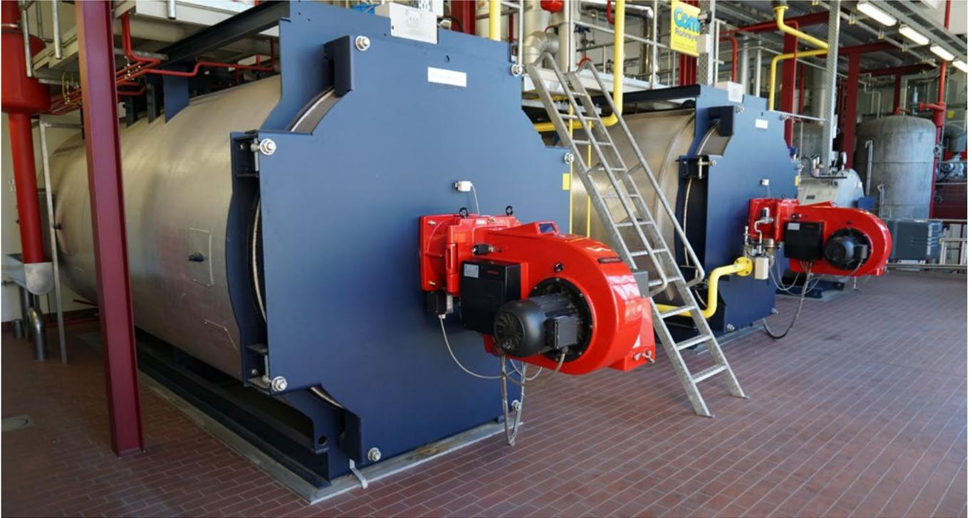
Two UNIMAT UT-H boilers generate a heat output of 7,000 kilowatts, and a UL-S UNIVERSAL steam boiler generates 1,250 kilograms of steam per hour.
