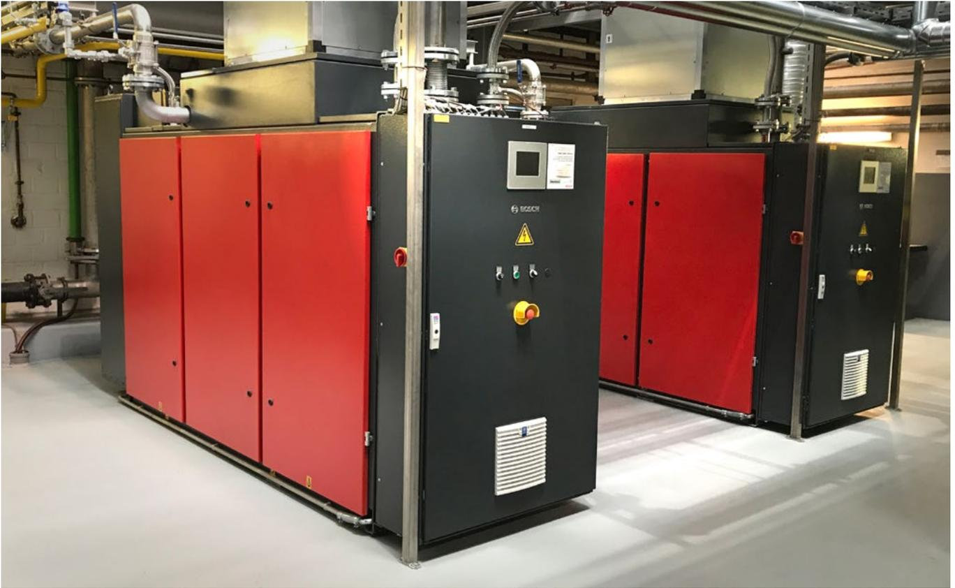
*Each of the compressed air and heat systems produces approximately 9.5 m<sup>3</sup>/min compressed air and 135 kW heat.*
