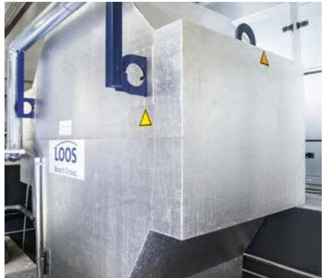
Separate flue gas heat exchanger connected downstream of the fourth smoke tube pass to provide maximum efficiency.
