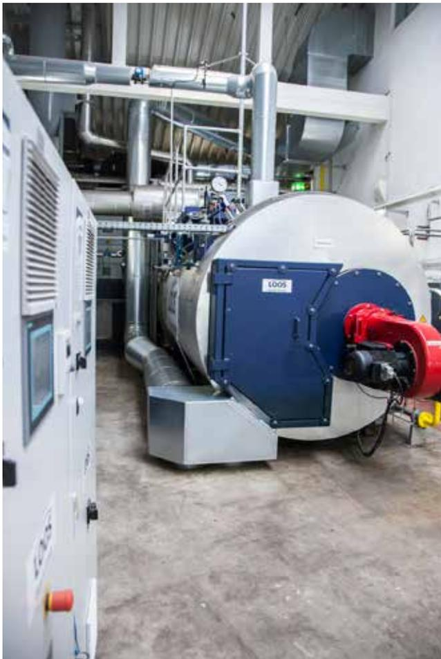
Maximum level of efficiency: the innovative boiler system with an additional fourth smoke tube pass and own firing.
