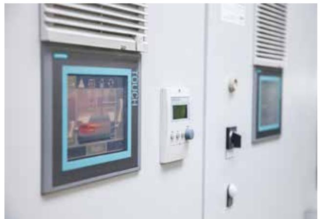
The modern BCO and SCO touchscreen controls enable the optimum setting and control of the boiler system.
