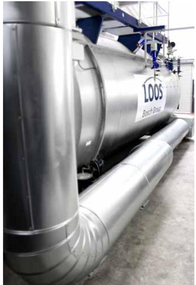
The additional smoke tube pass converts the waste heat from the CHP unit into process steam.
