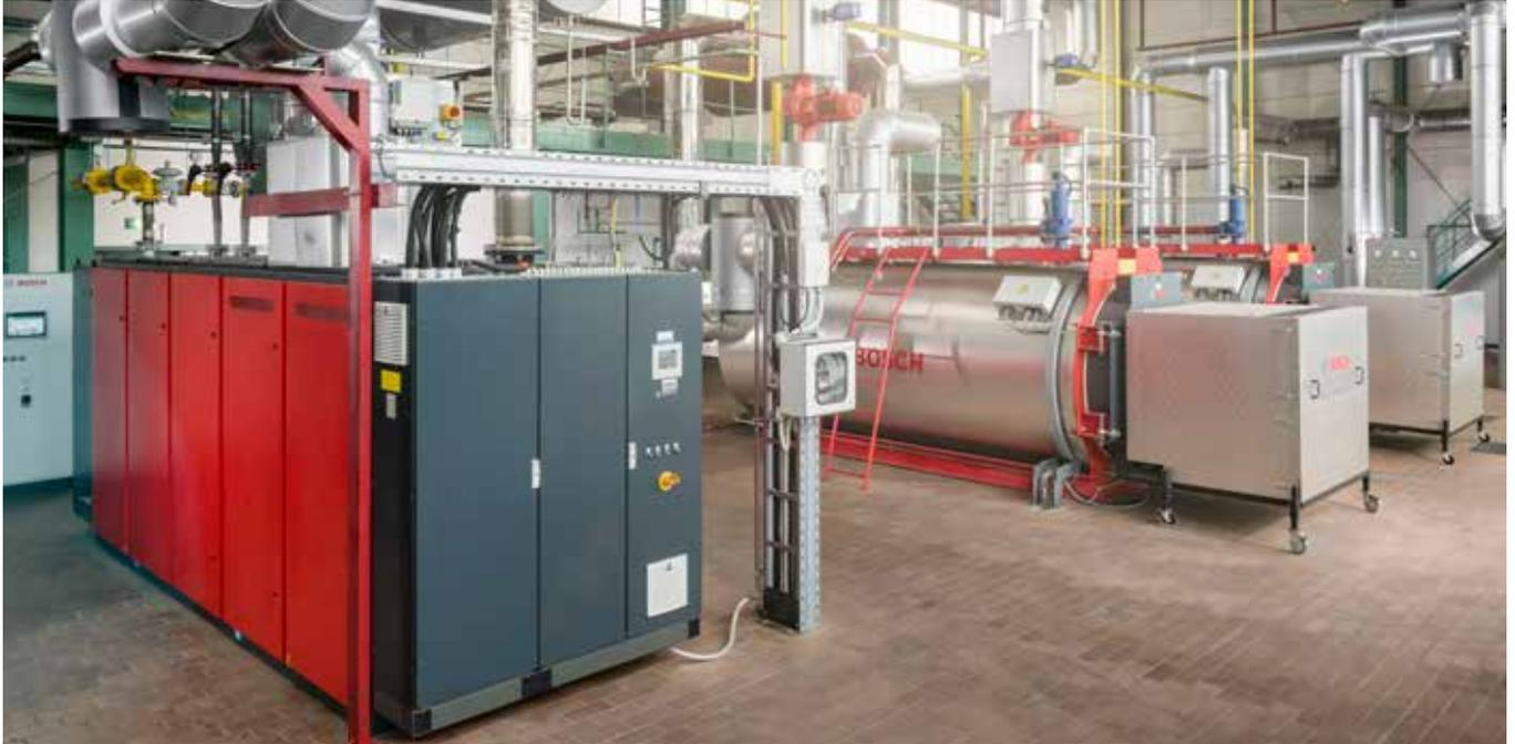
*The Bosch CHP provides the base load for heating and at the same time electric power for the company's own consumption.*
