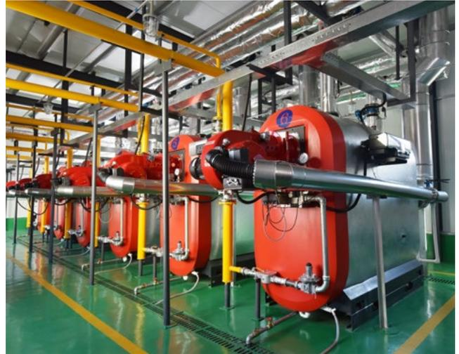
*Part of the Uni Condens heating boiler systems from the first order in 2016 – each boiler generates 1.2 MW heat.*
