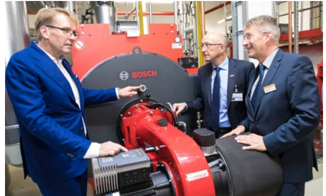
Strong team: Sven Koss of the executing planning office Koss Ingenieure together with Sven Evert, Bosch Industriekessel and Rainer Harms, Weishaupt.
