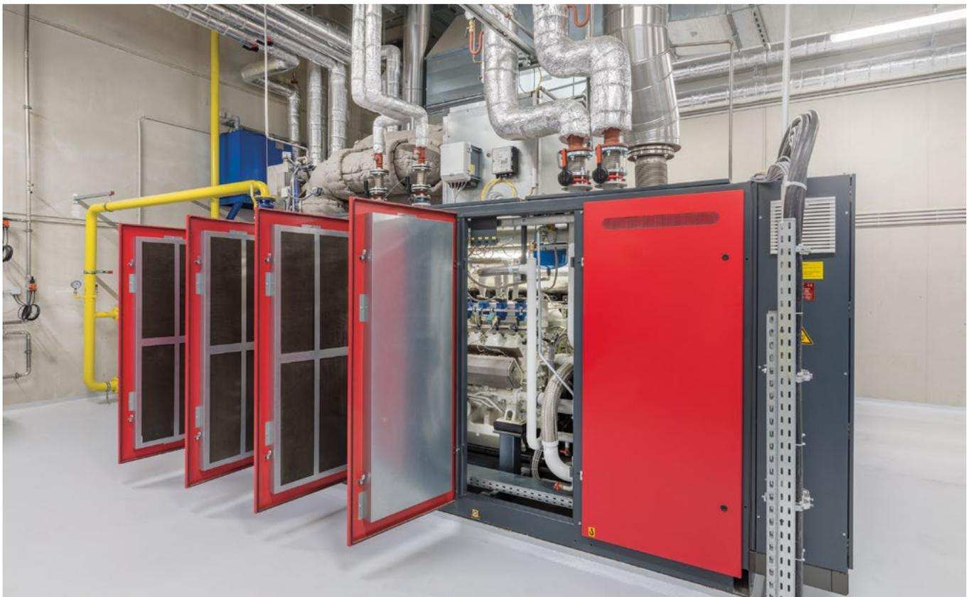
*The Bosch CHP system supplies the site with 400 kW of electrical and 500 kW of thermal output for power, heating and cooling.*
