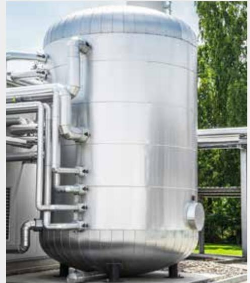
*The waste heat from the compressors and cold stores is buffered in the heat storage tank.*
