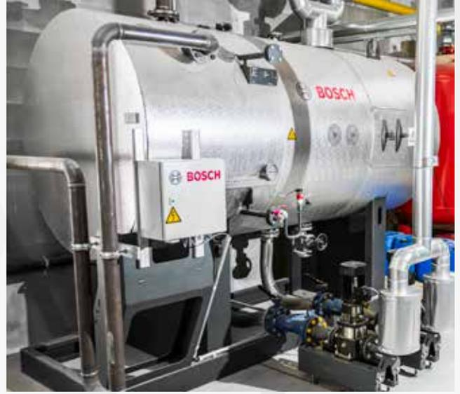
*Reduction in make-up water quantities through use of condensate service module.*
