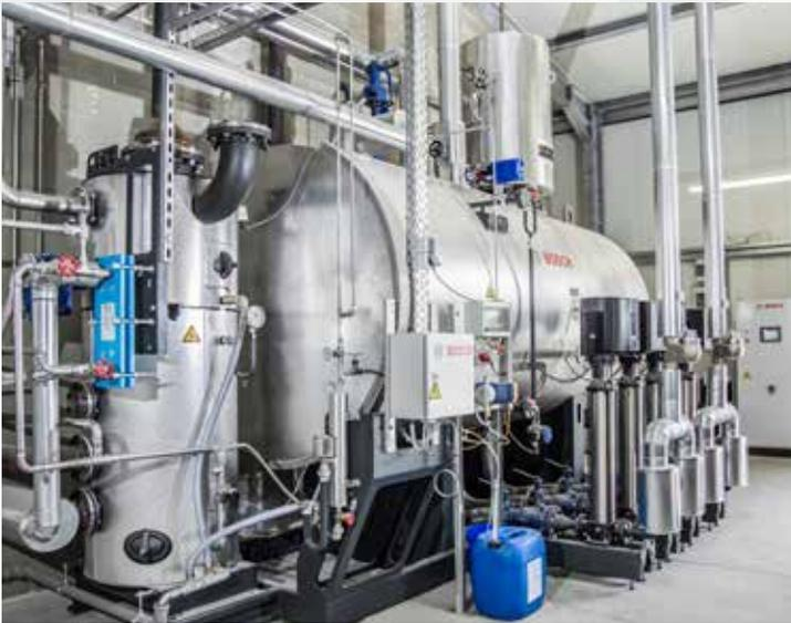
*The water service module with heat recovery from the desalting water.*
