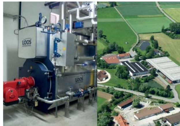
The U-MB steam boiler with SUC automatic start-up control at the beverage company Bissinger Auerquelle.
