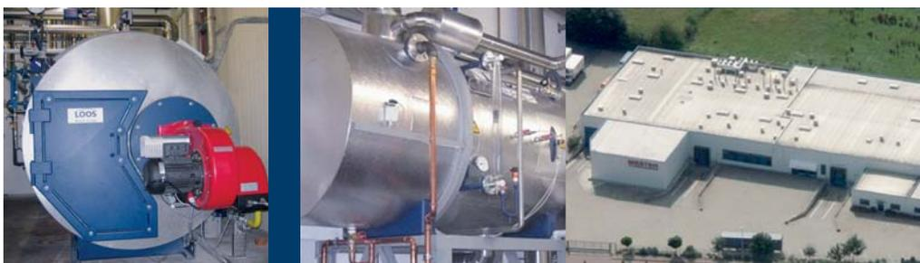
The Loos UL-S steam boiler with its innovative automatic start-up function and the feed water partial deaeration plant at the factory of Mester Altländer Fleischwaren GmbH.
