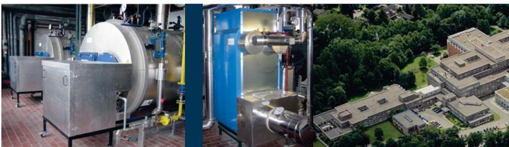
The state-of-the-art Loos steam boiler system with downstream stainless steel condensing heat exchangers ensures efficient energy supply at Itzehoe Hospital.
