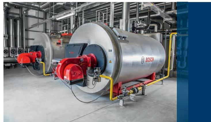
The modern Universal ULS steam boilers with modulating, speed-controlled natural gas burners
