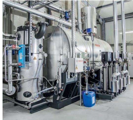
The water service module with heat recovery from the desalting water
