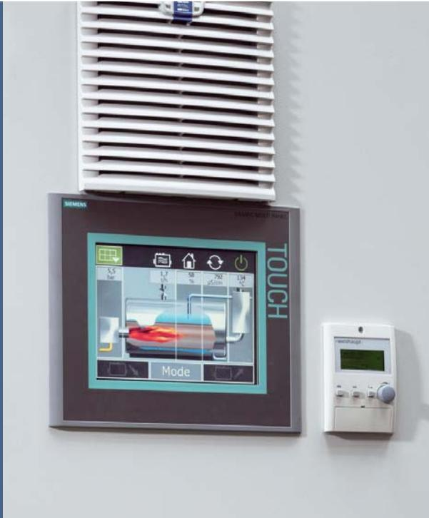
The operator also receives a swift and cost-effective solution to malfunctions via the tele-service in the BCO boiler control. Other system equipment includes an integrated economizer and dual firing for economic and environmentally-friendly operation. The boilers are fired with either natural gas or light fuel oil.
