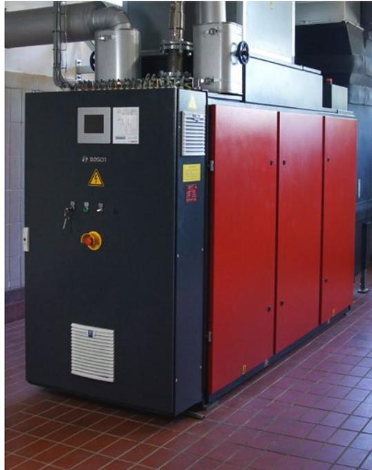
Operating for around 6,000 to 6,500 hours a year, the compressed air and heat system at Bahlsen covers the company's base-load need for compressed air.
