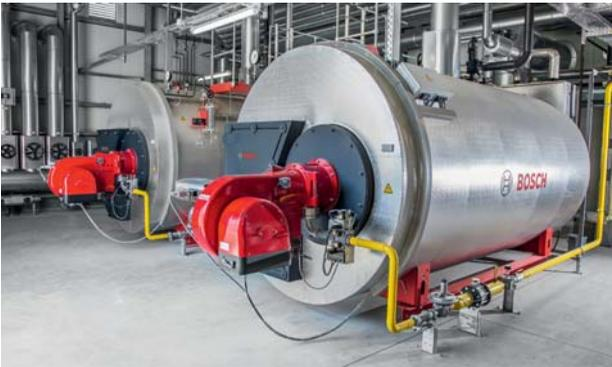
The highly efficient Bosch steam boiler system with speed-controlled natural gas firing systems.
