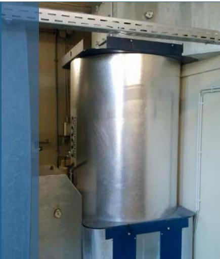
The retrofitted economizer makes efficient use of the energy from the hot boiler flue gases.
