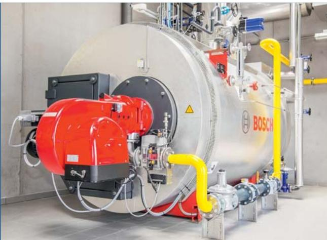
The state-of-the-art Bosch steam boiler efficiently provides the process heat for the production of animal feed.
