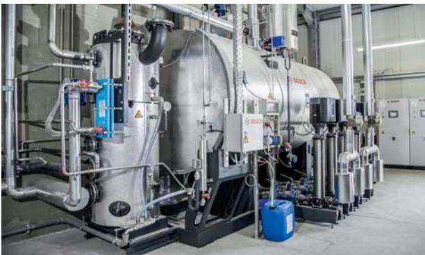
The WSM-V water service module provides the steam boilers with treated feed water. The integrated EHB heat recovery module uses the thermal energy from the hot desalted water.
