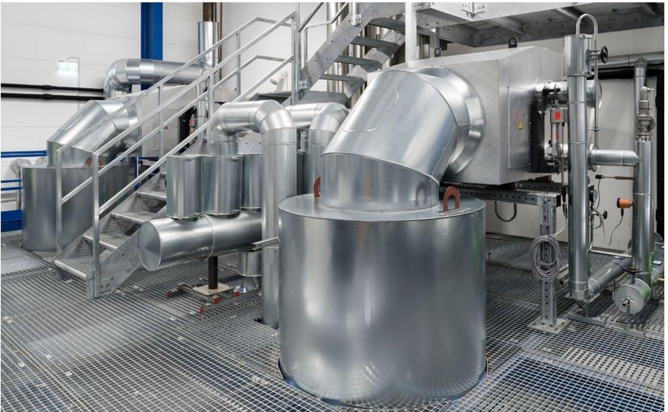
Condensing heat exchangers: Preheat process water cost-effectively with condensation heat.
