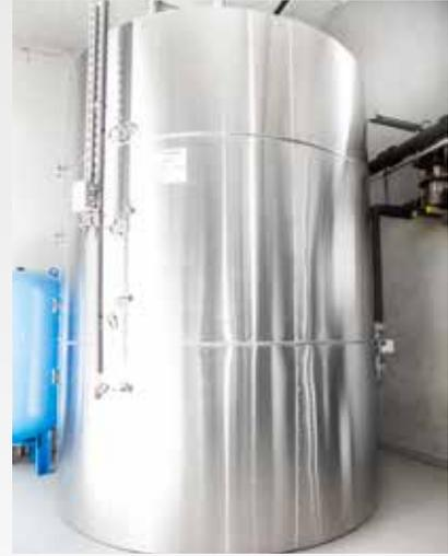
causing hardness (calcium and magnesium) from the raw water and forwards it to an osmosis plant for desalting. The softened water is pressed through a membrane at high pressure. The majority of the salts and other substances are left behind and the pure water that exits the membrane is fed into a heat storage tank with a capacity of 6,000 litres.
