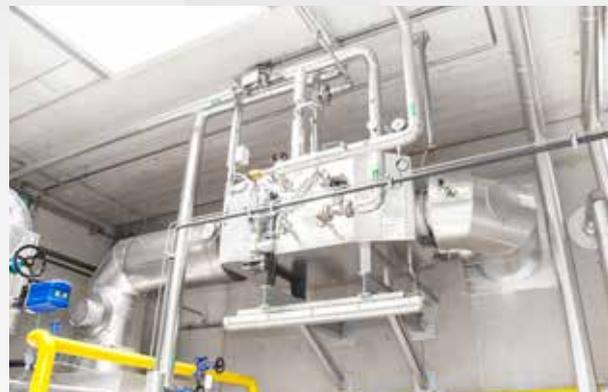
*The condensation heat from the condensing heat exchanger (image) and the heat from the exhaust vapours heat up the make-up water prior the deaeration process.*
