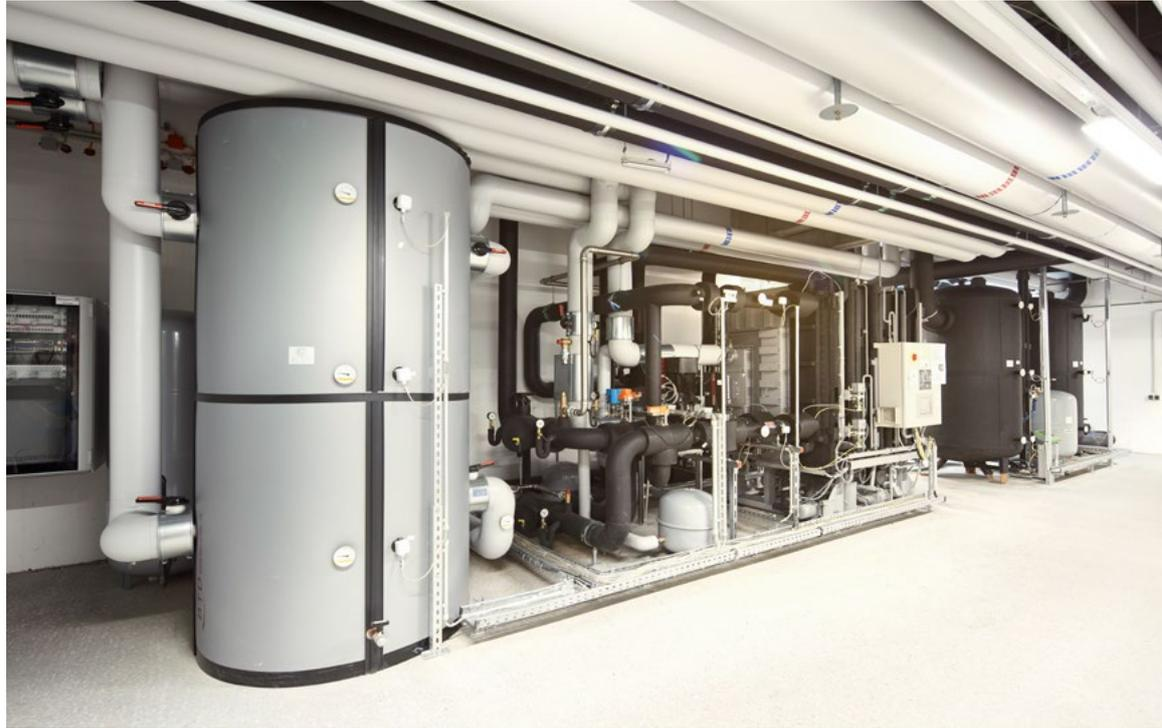
buffer tank allows the CHA higher annual running times as the heat can be temporarily stored. An additional 800 kW is supplied by a SB745 boiler of the Bosch brand Buderus.
