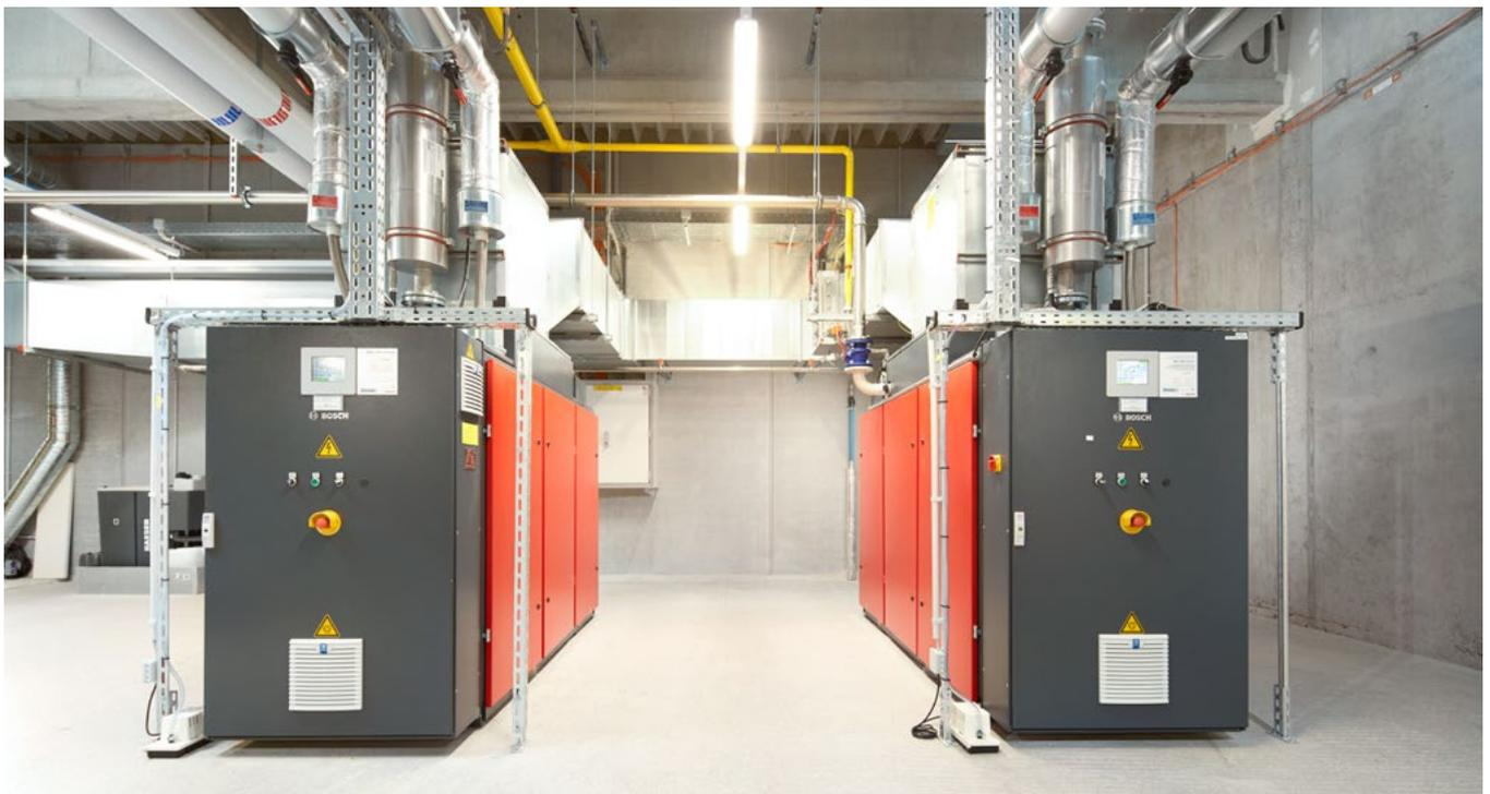
*The two compressed air and heat systems from Bosch supply the company building with the base load requirement of compressed air of 17.5 m<sup>3</sup>/min and 250 kW heat output.*
