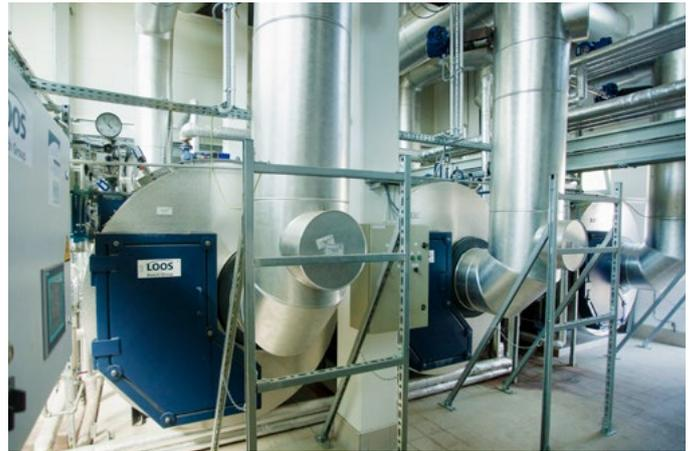
The waste heat boilers use the CHP waste heat for cost-efficient steam generation.
