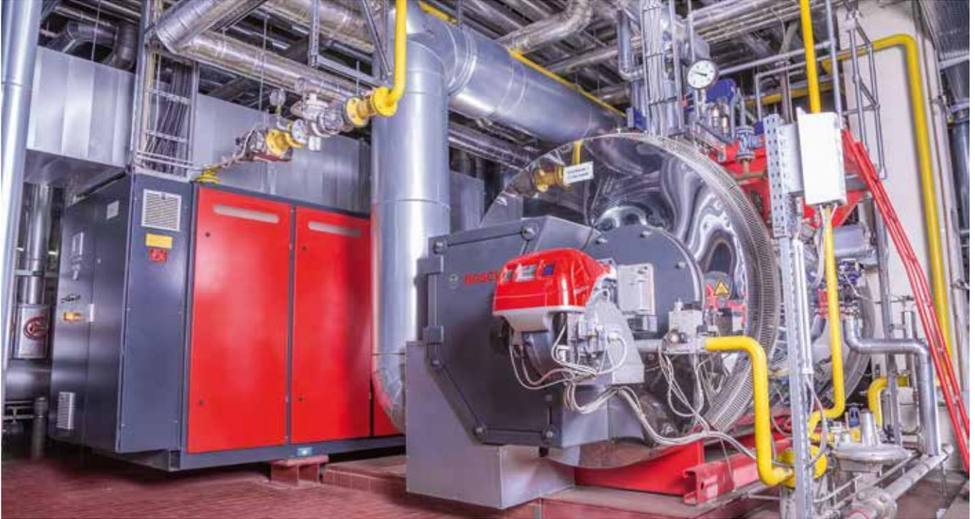
*Effective use of waste heat sources: The CHP waste heat with temperatures of up to 550 °C are passed through the fourth pass of the steam boiler and used for the steam generation.*
