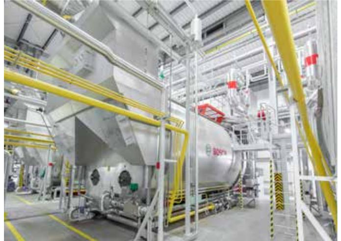
Top-mounted Economiser for unlimited individual use of burners. The individual operation of the burners is therefore permissible.
