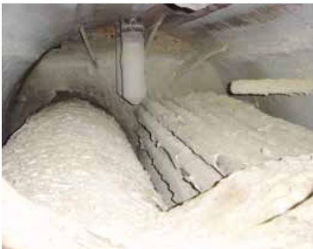
Figure 1: A lack of water treatment caused the formation of a hard layer which can lead to boiler explosion in the extreme case.
